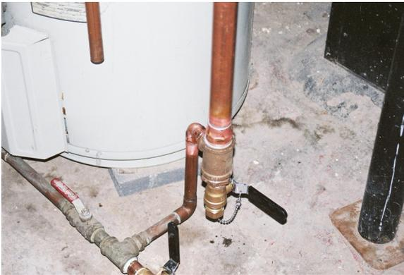
I removed the anode rod from my tank and installed a galvanized nipple and cap in its place.
