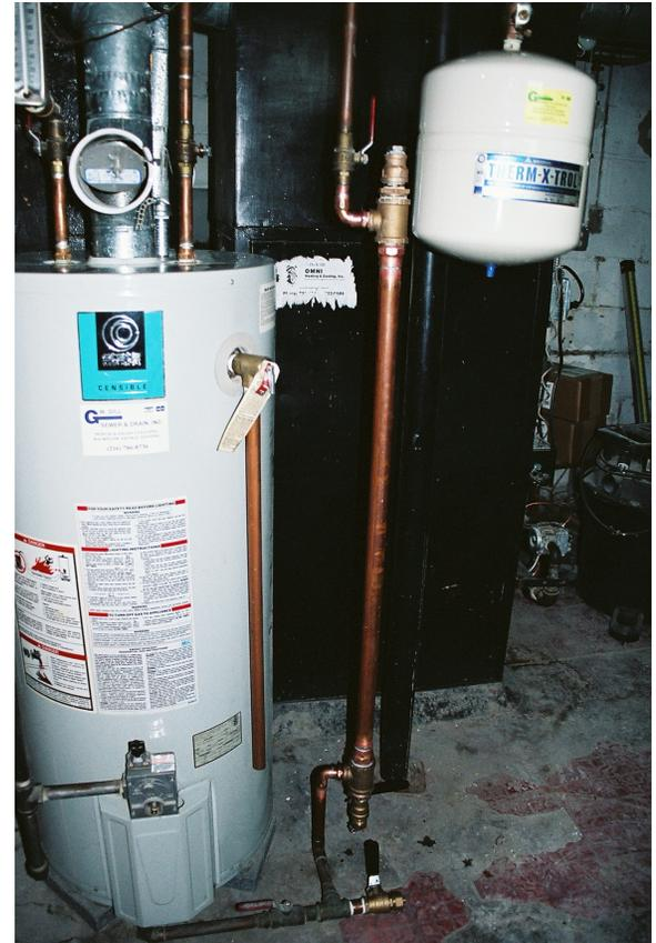
Presently there is no corrosion evident at any bimetal tank connections on the top of the tank and only slight discoloration at the T&P boss. The experiment calls for the inspection of the anode at regular intervals to determine rate of decay and to visually inspect tank connections for corrosion.
