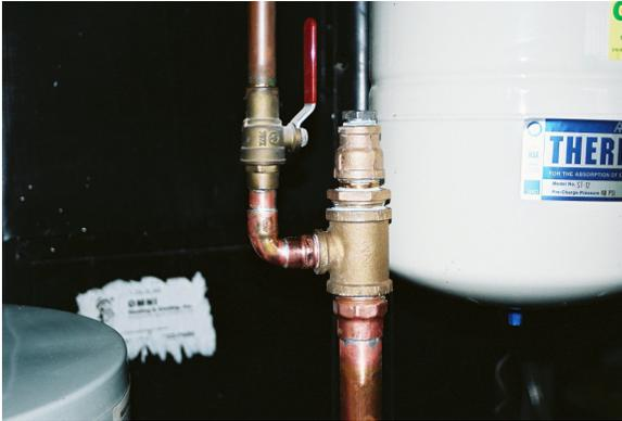
Background- Due to some water heater brands having an anode rod that is combined with the hot water outlet nipple, a question arose in my mind as to whether an anode placed in a chamber exterior to the tank would still provide cathodic protection to the tank. If it were to work it would provide extended water heater life by making it easy to replace the anode rod at periodic intervals.
